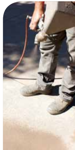
Hopper gun application of Stylepave.
